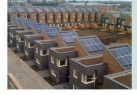
AccuRoof from SIG Roofing has specified an innovative SolarNature biosolar system in partnership with Eco Green Roofs. The green roof element supports the photovoltaic panels' operating temperature envelope, and the PV's wind and sunshade help improve the diversity of vegetation. As a result, the biosolar roofs contributed positively to the Urban Greening Factor ("UGF") of developments in 2022 and 2023.
