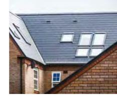
THE SOLUTION As the housebuilder had used Cembrit Moorland slates before, they decided to specify the product range on this housing development in Abergavenny. Main contractor, Avonside Roofing, installed the slates on a design that featured pitches ranging from 35° to 57°, and also consisted of dormer windows, vents, verges, hips,
