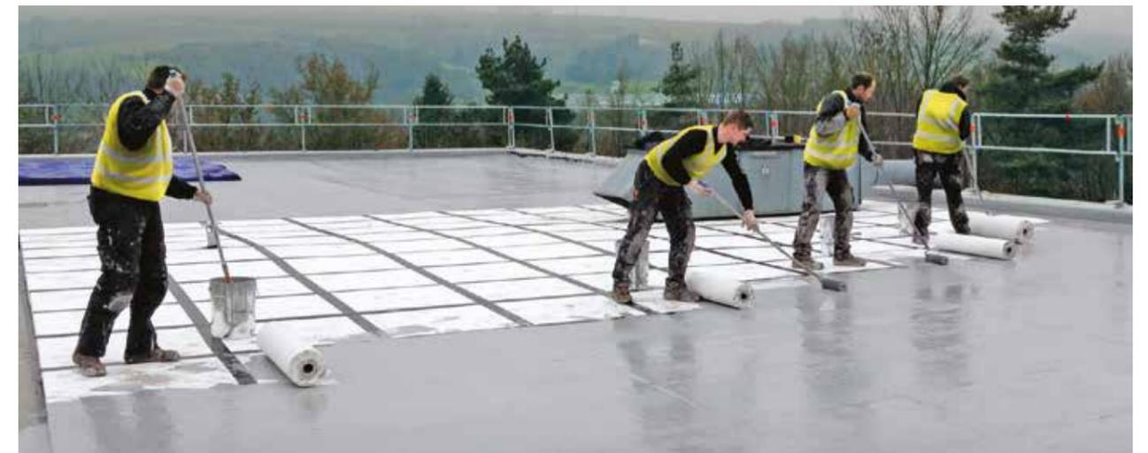
Before you apply liquid waterproofing, there are three essential steps to ensure a top-notch job: planning, preparing the surface, and priming areas as necessary.
