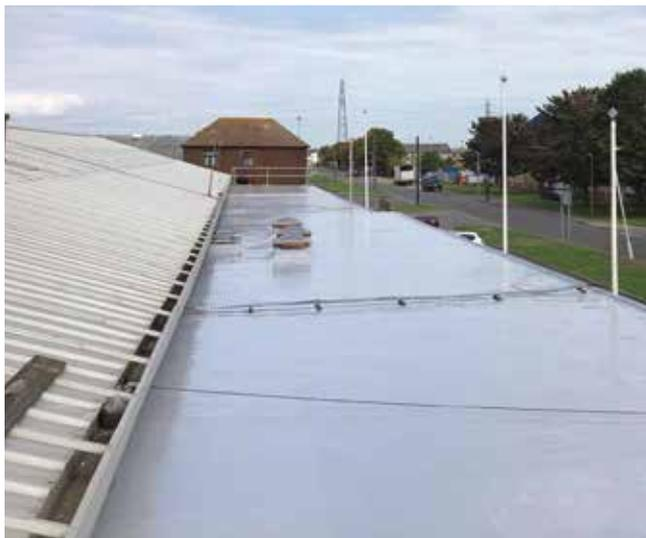
Create a durable and seamless light grey waterproof layer, in a single coat, with PU-10 Liquid Coating.
