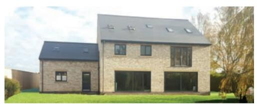
Durham-based roofing contractor, Wilkinson Roofing installed approximately 3,000 600x300mm Cembrit Jutland fibre cement slates on the roof of the house and garage. Their aesthetic appeal and proven performance were key factors in the specification.
