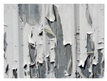
Knowing the tell-tale signs of cut edge corrosion can save you and your customers a lot of trouble. When the steel or aluminium sheets used in metal cladding are coated with a protective layer of plastic and cut to size in the factory, the cut edge isn't coated as part of the process, leaving the material prone to corrosion and coating failure.
