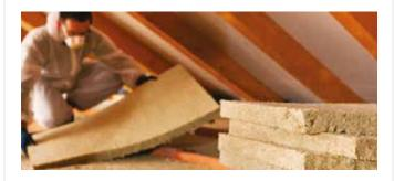
When upgrading the levels of insulation in a roof space, it is important to ensure that the existing levels of roof ventilation are adequate.
