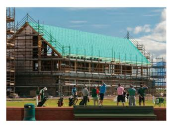
and vapour permeable. Recognised as one of the highest performing roofing membrane solutions, it has become the preferred choice of architects, developers and contractors. Tony Bowe site manager for Ogilvie Construction explains his reasons for the selection of Roofshield. "We chose Roofshield because of its superior quality and breathability, assuring protection for the new buildings at Carnoustie."
