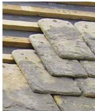
Traditional Slate Peg Fixing
