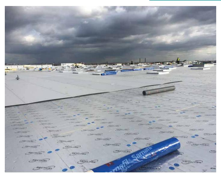
Ideal for warm flat roofs as part of a mechanically-fixed, single-ply membrane system, Eurothane Eurodeck is a high-performance, rigid PIR foam board with exemplary environmental credentials:
