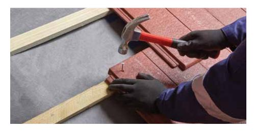
it looks like one of its small format cousins, while its double tile format has a mock joint giving the appearance of small tiles when laid broken bonded. Russell have also introduced three other thin leading edge concrete tiles, the Lothian, Moray and Polden to ensure you can find an appropriate alternative to traditional slate or clay.
