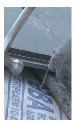
Traditionally, clips and nails come in separate bags and need threading together before installation, which adds to labour time and cost. As a one-piece clip and nail, SoloFix, comparable in price to standard aluminium clips, can save contractors as much as 30% on roof clipping time.
