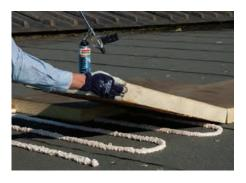
Soudatherm Roof Adhesives Soudatherm Roof Adhesives are ready-to-use liquid polyurethane adhesives that bond insulation materials – such as extruded polyurethane foam, polystyrene, phenolic foam or mineral wool – onto horizontal surfaces, aged bituminous roofing membranes, etc. All variants:
