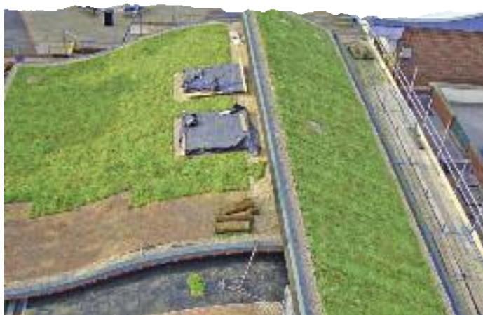
Single-layer insulation systems are also perfect for green roofs.
