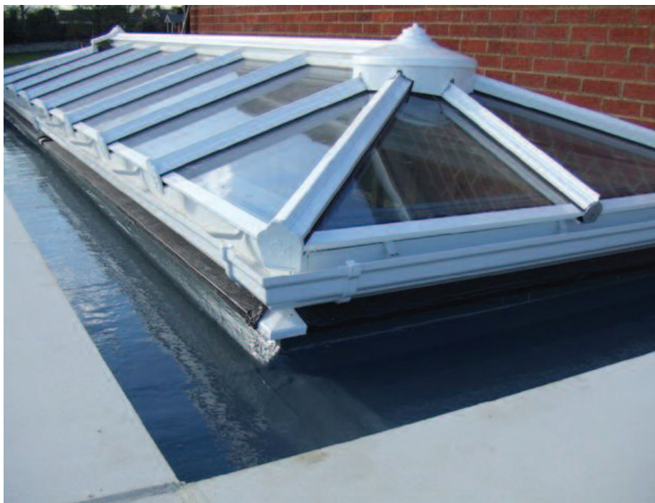
CrysticROOF is cold GRP system, which comes with a 10 Year warranty from Scott Bader. It is suitable for flat roofs, valley, pitched and complex roof designs.
