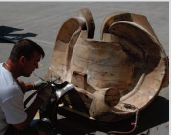
The lion heads all appear to be identical from a distance, however upon viewing close up it is clear that each mouth and jaw are slightly different. This meant that the cutting and shaping for each was individual and not from a one off template. Four leadworkers were given the task of completing two cartouches with each cartouche taking 10 days of solid and exacting workmanship.
