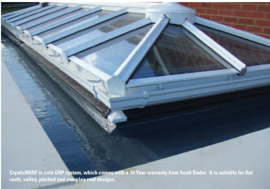
CrysticROOF is cold GRP system, which comes with a 10 Year warranty from Scott Bader. It is suitable for flat roofs, valley, pitched and complex roof designs.
