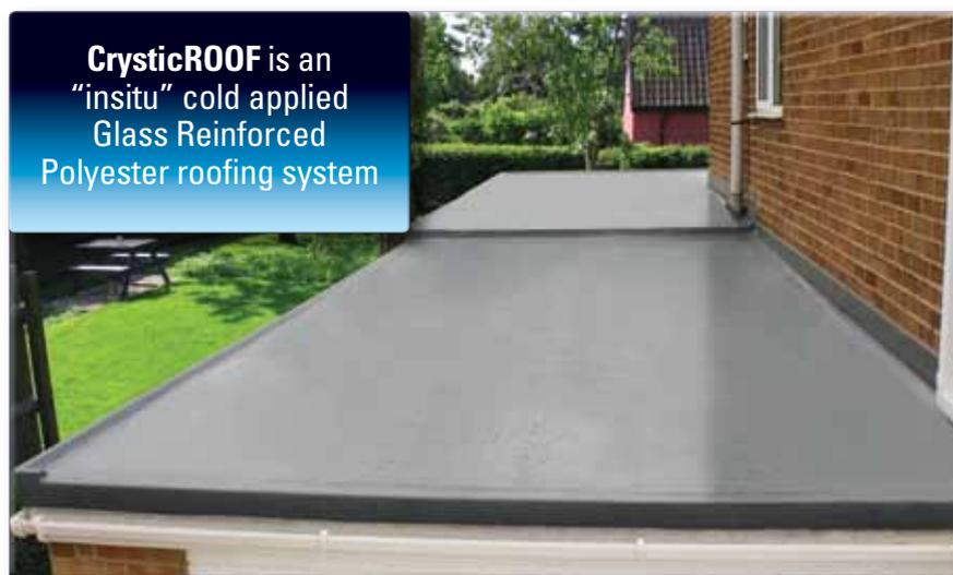
**CrysticROOF** is an "insitu" cold applied Glass Reinforced Polyester roofing system
