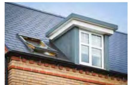
loft windows, dormers, and abutments. This process provides wind uplift resistance, which helps in creating a long-lasting roof covering. We also installed Cembrit low profile roof slope vents for adequate ventilation. The Cembrit slates were extremely easy to cut and fix, and we are extremely pleased with the end result."
