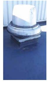
Working around various extractors, air conditioning units and pipes, the threeman team tackled the roof in sections, laying and taping a new timber deck, painting it with FG Alutrix Primer. An Alutrix 600 vapour control layer followed, with IKO Enertherm Alu Faced insulation fully adhered on top. The ready to use, cold-applied top coat of FIX-R Liquid Waterproofing is vapour permeable, giving the restaurant roof resistance to standing water, UV stability and no shrinkage.
