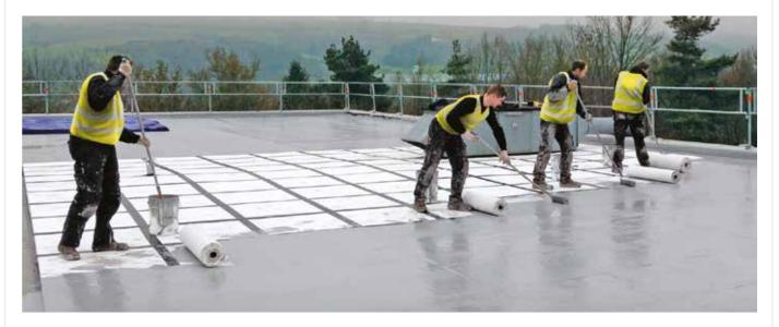
Before you apply liquid waterproofing, there are three essential steps to ensure a top-notch job: planning, preparing the surface, and priming areas as necessary.
