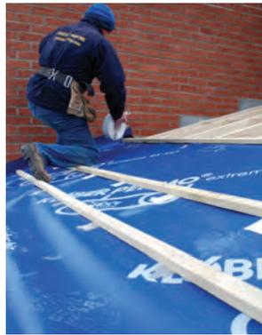
fleece which allows vapour to escape, while keeping water out.
