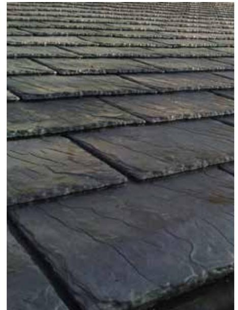
Over time the slates self-bond to form a solid membrane on the roof that is wind and weather resistant, even at low pitches. This process relies on sunlight, bonding even quicker during the summer.
