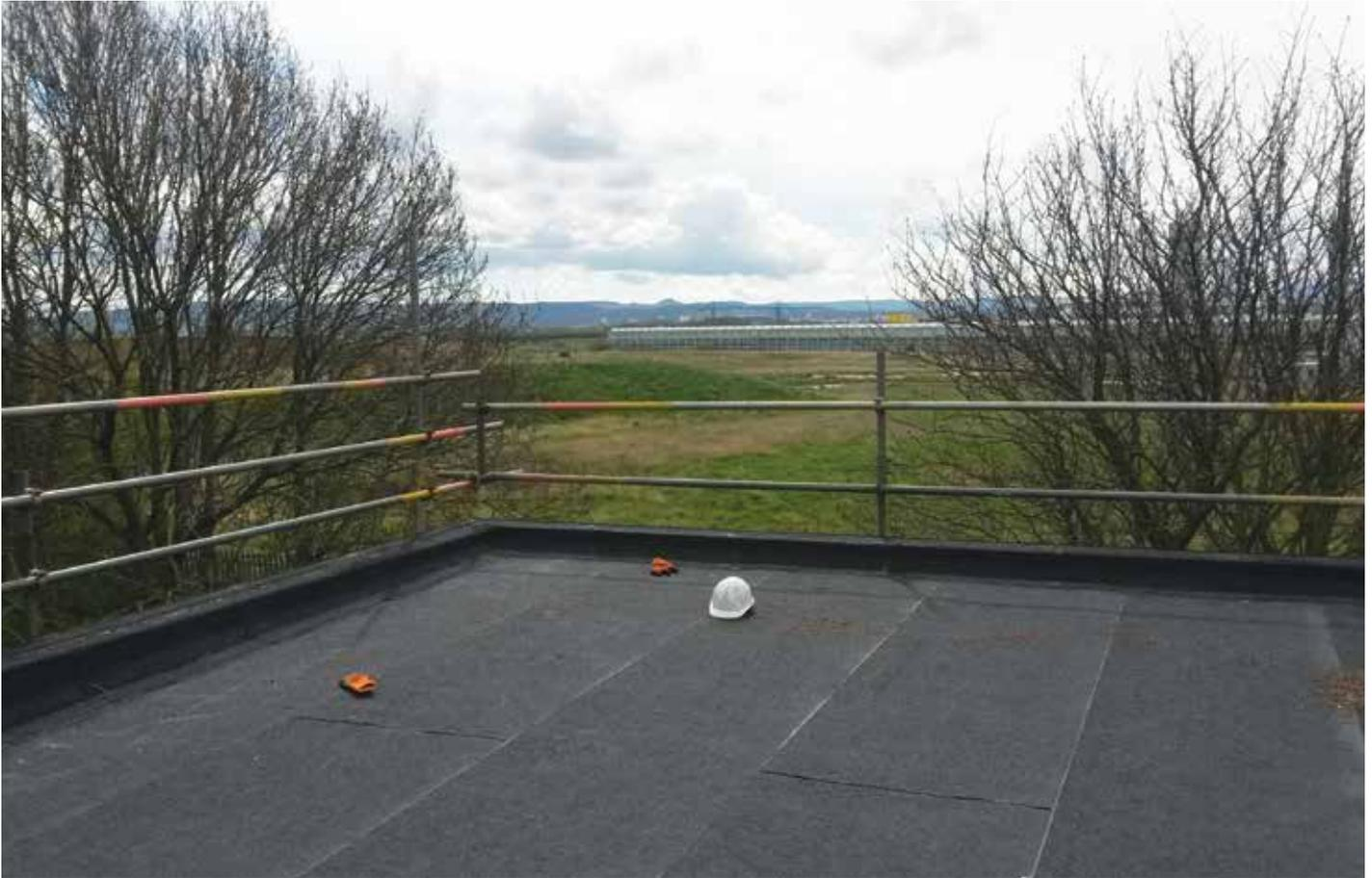
DVC Roofing won the contract and work began in May 2016, with the first task being to prepare the site safely. As part of that the factory was fully netted, both to protect the contractors from falling and shield the factory workers from falling debris. The existing defective materials were then stripped back to the metal profile sheet. All the old flat roof skylights were removed and replaced with new barrel vaulted insulated aluminium windows.
