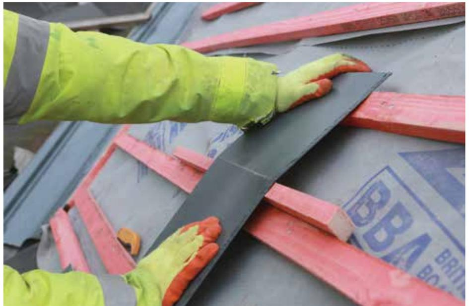
you can cut them by hand on site is just one of the reasons they are becoming so popular. For example, Marley Eternit's range of fibre cement slates are available in uniform size, shape and thickness, and can all be scored and snapped, or cut with a guillotine or reciprocating saw. It makes them very quick to install without the need for water suppression.
