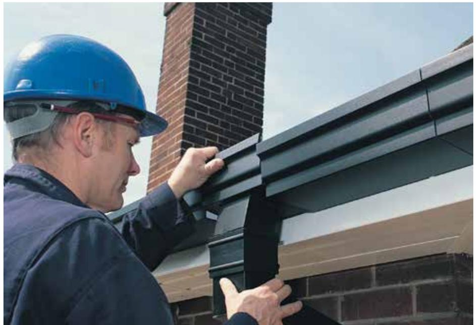
As well as improving safety, aluminium's reduced weight can also save you money. Being so easy to handle on site, aluminium systems are generally quick to install and take fewer tradesmen to do the job. It means you can complete more work, faster, and get a head start on the next project. Aluminium systems also offer impressive performance with the best boasting life expectancies of 50 years or
