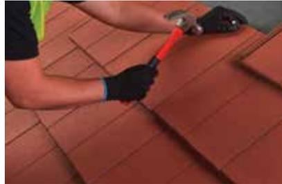
Bute is the latest addition to the Natural Range of concrete tile versions of slate, clay and stone – each designed to match the local look of roofs across the UK. It has a double tile format, so has the good looks of a small format tile, however it's easier to fix. One tile covers a larger area but still has the appearance of smaller tiles, which means you'll spend less time up and down the ladder and more time admiring your handy work.
