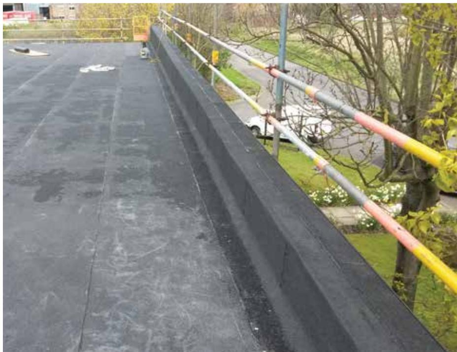
caused by high humidity inside the building, exacerbated by a lack of ventilation and the cold roof design were all contributing factors to the roof's condition.
