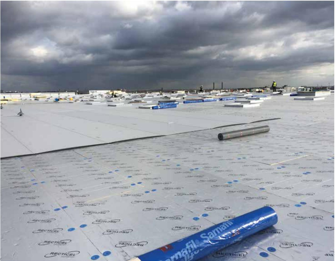
**Ideal for warm flat roofs as part of a mechanically-fixed, single-ply membrane system, Eurothane Eurodeck is a high-performance, rigid PIR foam board with exemplary environmental credentials:**
