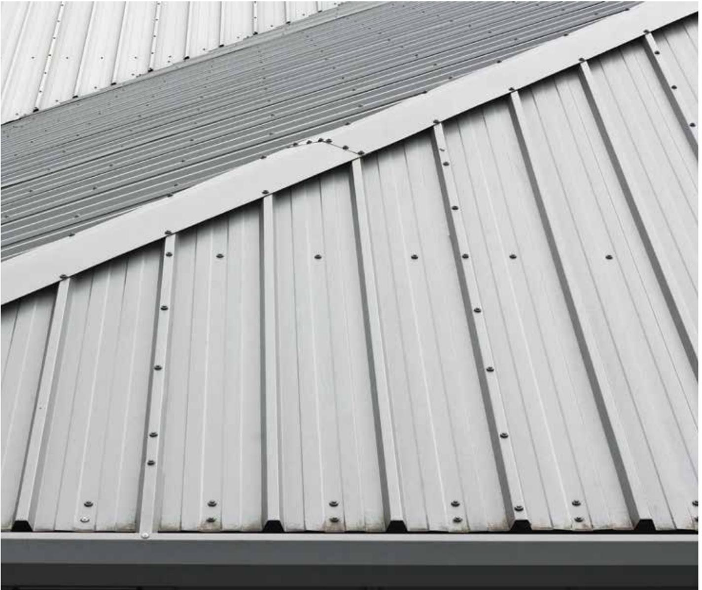
Another cause is the changing shape of the metal substrate. Metal can expand with rises in temperature and contract when cool. As the cladding expands, the factory coating can lift which exposes the underlying substrate. Consequently, the elements take their toll and eventually more and more of the coating can delaminate.
