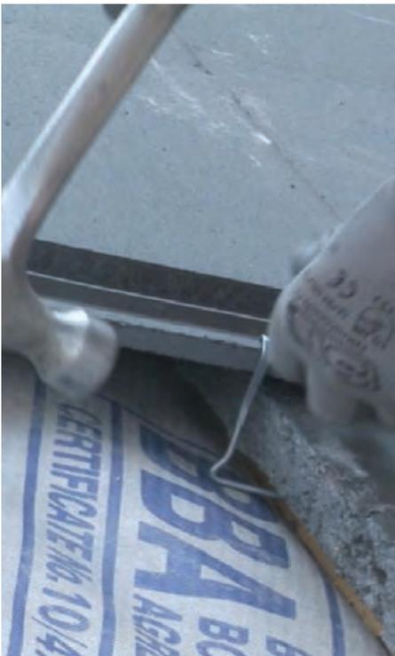
Traditionally, clips and nails come in separate bags and need threading together before installation, which adds to labour time and cost. As a one-piece clip and nail, SoloFix, comparable in price to standard aluminium clips, can save contractors as much as 30% on roof clipping time.
