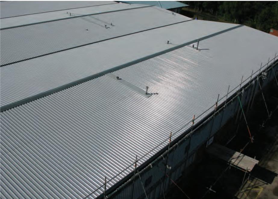
When the existing asbestos cement roof started to fail at Coleg Cambria, Wrexhams' higher education college, Filon over-roofing was used to refurbish the Engineering Centre of Excellence.
